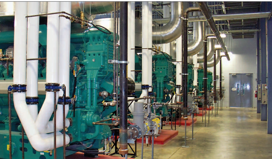
LEFT Five Cummins Power Generation generator sets — four gas and one diesel — installed at a hospital. RIGHT This paralleling switch from Generac Power Systems allows the main power leads of each generator to be connected together at a common point.
