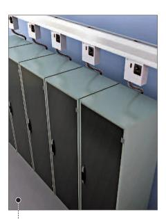
**HANDY SOLUTION** The Track Busway system offers one-handed operation to add or remove outlet boxes or drop cords quickly and easily without cutting off power to the entire busway. It also features one soldered connection that increases savings with reduced parts, long product life and fewer failure points.
