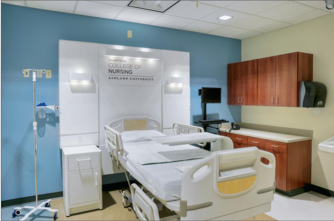
**HEADY SOLUTION** The headwall system features modular, removable panels that can be adapted easily to changes in technology and are made primarily with a nonporous DuPont Corian surface for added durability. Leads, gas taps and other medical equipment are concealed from patient view to provide a more relaxing environment. **Futrus Solutions • [www.futrus.com](http://www.futrus.com)**
